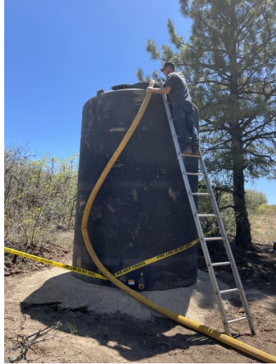
5,000-Gallon Tank set in place
